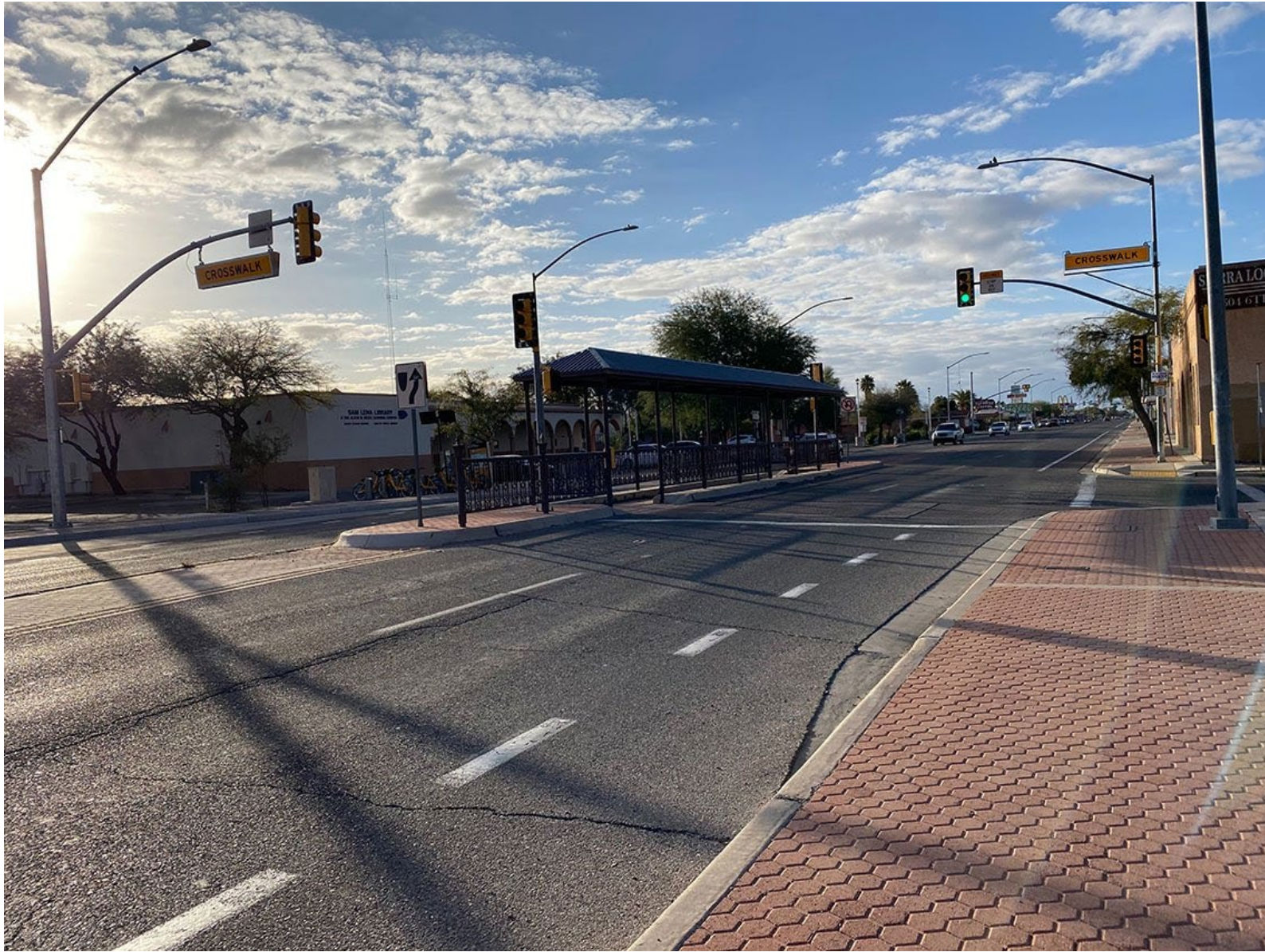
Image: Major street and sidewalk without separation from the roadway (not detached)
