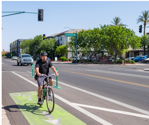
The use of additional pavement markings delineates space between vehicles and bicyclists.
