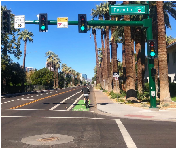
Buffered bike lanes should include a striped buffer that is at least 2.5-3+ feet
