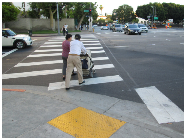
Not recommended: Diagonal curb ramp configuration.
