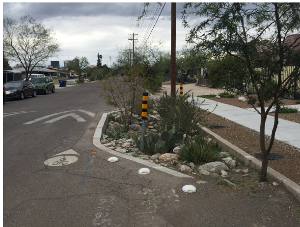
Bulb outs narrow the right-of-way, creating visual friction and slowing cars.
