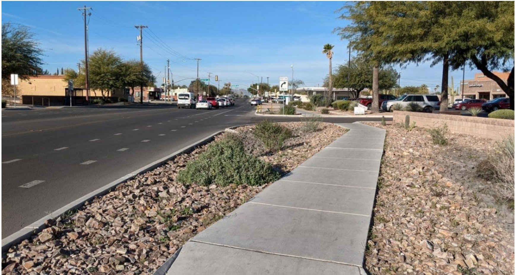
Image: Major street with detached sidewalk
